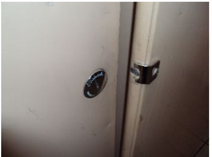
Toilet partition door doesn't latch (Mens Locker Room)
