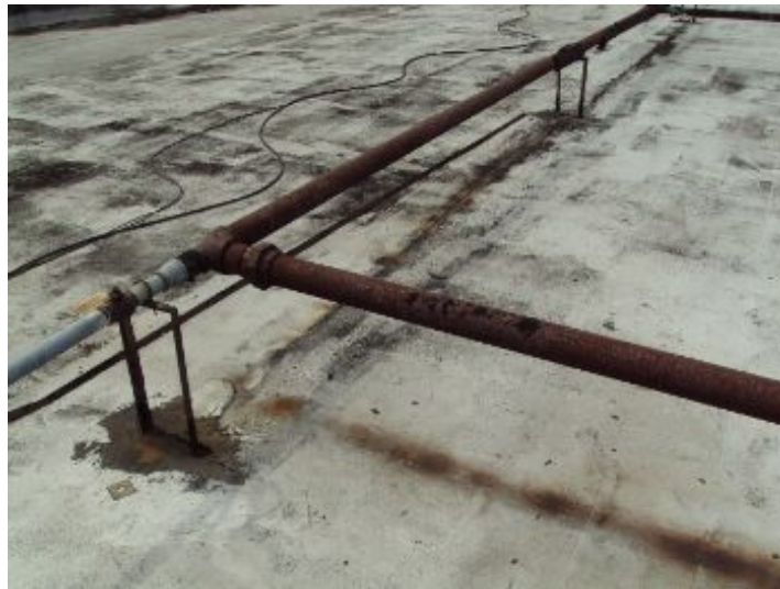
Scrape and paint gas piping at the roof
