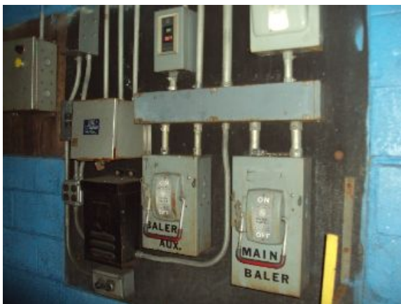
Baler controls not energized at the time of inspection
