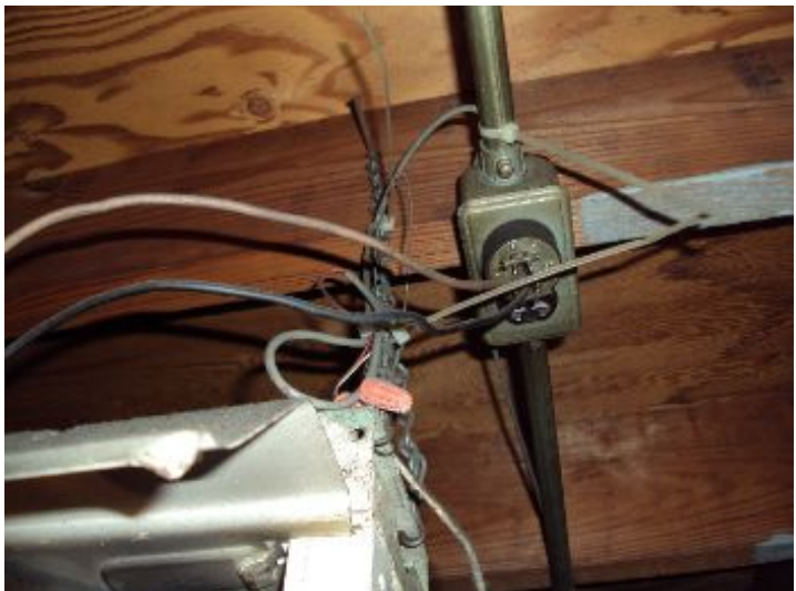
Improper wiring
