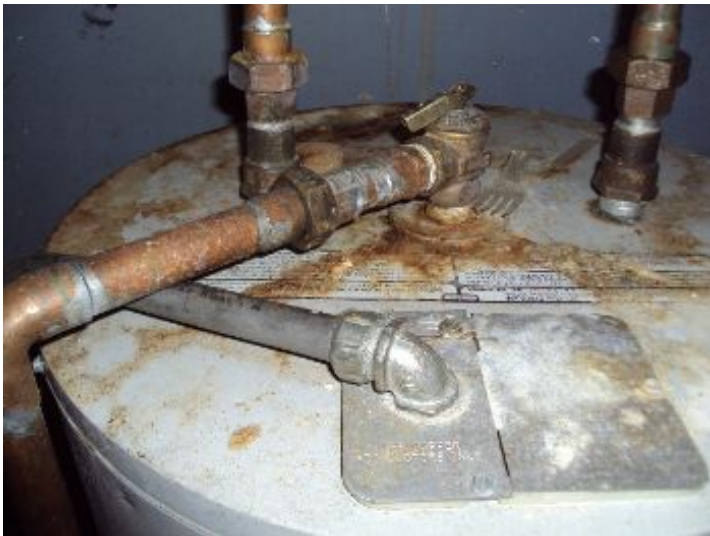
Prior leaks and deterioration
