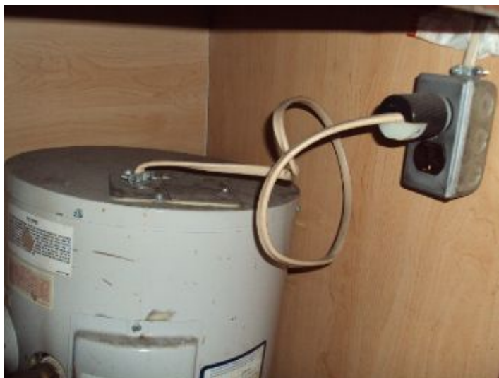
Cord connected water heater.
