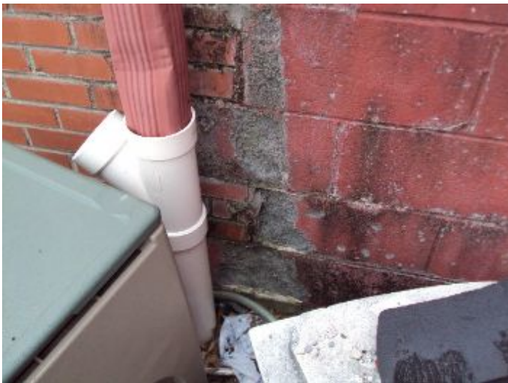
Severe spalling
